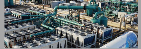
Lightning Dock geothermal power plant in the Animas Valley
